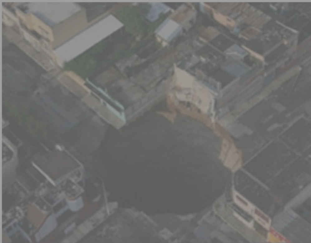
A sinkhole in Guatamala
